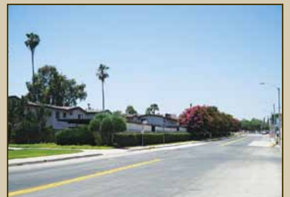
A look at the newly completed Mission Road, with new subgrade, two layers of asphalt, and striping.
